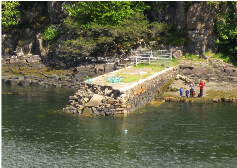
Aros Pier before
