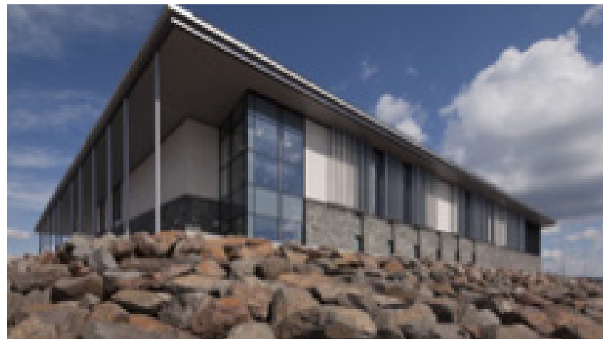
Improved Flood Defences – raised and extended Rock Armour, new sea wall, and raised ground levels across the site
