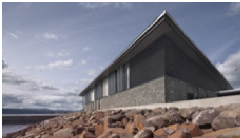
Improved Flood Defences – raised and extended Rock Armour, new sea wall, and raised ground levels across the site
